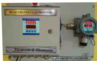
Gas Leak Detection System
